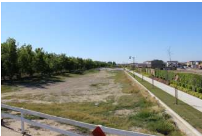
Mooney Blvd. currently ends at Shannon Pkwy, but should eventually connect to Riverway Dr. & Pratt Rd.
